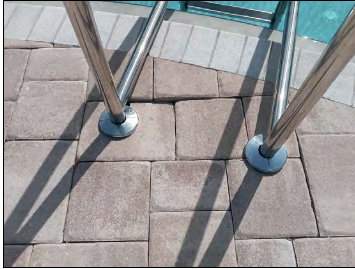
Sinking pavers at one of the pool stairs.
