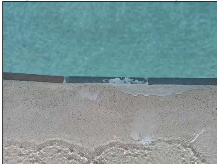
Some type of white mineral deposit is occurring at the tops of the tile on the shelf around the perimeter of the pool.
