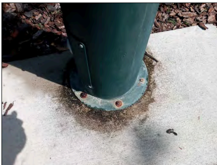
The drinking fountain by the playground is leaking from within and there is a white deposit in the bowl and down the side of the fountain.
